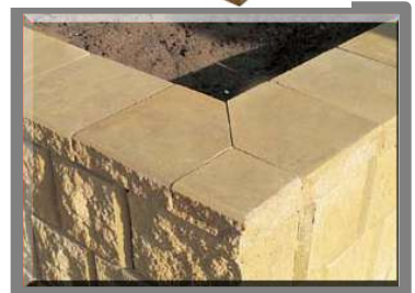
Internal Corner Caps - Cutting Detail
